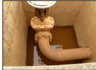
Sumps, Wet Pits, Catchments
