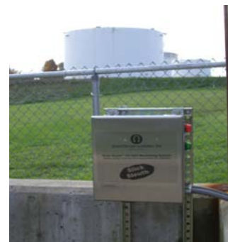
Figures 17, 18 & 19. Typical applications - sensors used for monitoring cooling water and storm water discharge for varying types of oils that could be spilled at refineries, power plants, and tank farms respectively. Alarm and data output sent in real-time to plants' 24-hr control room for instant notification and response. Note that Figure 17 (on left) depicts a unit housed in EXd-rated explosion-proof housing.
