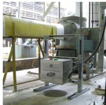
Figures 17, 18 & 19. Typical applications - sensors used for monitoring cooling water and storm water discharge for varying types of oils that could be spilled at refineries, power plants, and tank farms respectively. Alarm and data output sent in real-time to plants' 24-hr control room for instant notification and response. Note that Figure 17 (on left) depicts a unit housed in EXd-rated explosion-proof housing.
