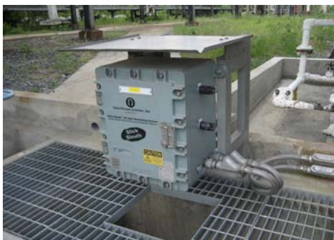
Figures 17, 18 & 19. Typical applications - sensors used for monitoring cooling water and storm water discharge for varying types of oils that could be spilled at refineries, power plants, and tank farms respectively. Alarm and data output sent in real-time to plants' 24-hr control room for instant notification and response. Note that Figure 17 (on left) depicts a unit housed in EXd-rated explosion-proof housing.
