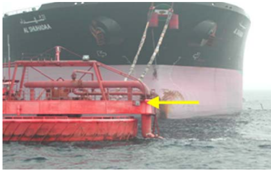
Figures 22 & 23. Spill sensors mounted on the outer circumference of offshore tanker loading buoys. 2-sensors mounted on each buoy at 180° (i.e. on opposite sides of buoy). Oil-on-water alarms are sent to shore side operations personnel in control room via radio link, then relayed to bridge of tanker vessel to provide near-instantaneous alert of oil spill occurrences.
