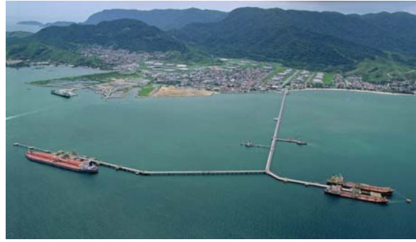
Figure 21. Array of spill detectors being deployed at this terminal, to monitor for both heavy-oils and lighter Benzene fractions. Sensors strategically placed at points along the piers. Local audio/visual alarms on pier plus wireless signal to control room.
