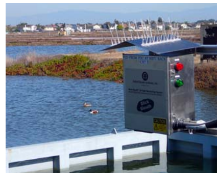
Figures 9, 10 & 11. Remote spill detection system (4-units total) used to automatically control tidal gates and alert personnel to incursion of oil in wetlands/tidelands near production area. Oil producer collaborated with the State of California to safeguard the Bolsa Chica Wetlands, a tidal zone with many valuable indigenous species.
