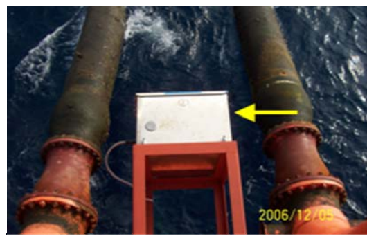
Figures 22 & 23. Spill sensors mounted on the outer circumference of offshore tanker loading buoys. 2-sensors mounted on each buoy at 180° (i.e. on opposite sides of buoy). Oil-on-water alarms are sent to shore side operations personnel in control room via radio link, then relayed to bridge of tanker vessel to provide near-instantaneous alert of oil spill occurrences.
