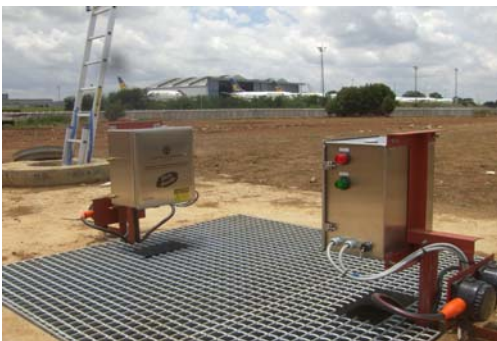
Figure 24. Sensors mounted above storm water discharge canals, monitoring for jet fuel or incidental diesel/oil in runoff from airport tarmacs. Detection alerts airport personnel to shut control valve between discharge canals under airport property, before subsequent outflow to public waterways downstream.
