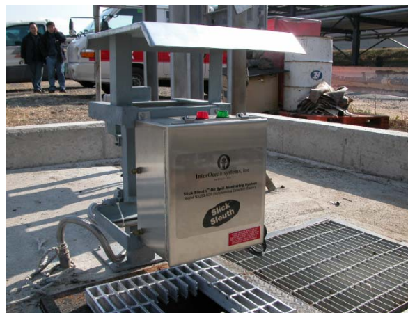
Figure 5. Oil detection sensor installed over discharge sewer at refinery. Real-time notification to facility personnel, night and day, around the clock, for all types of crude and refined oils.
