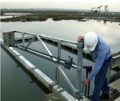
Figures 9, 10 & 11. Remote spill detection system (4-units total) used to automatically control tidal gates and alert personnel to incursion of oil in wetlands/tidelands near production area. Oil producer collaborated with the State of California to safeguard the Bolsa Chica Wetlands, a tidal zone with many valuable indigenous species.
