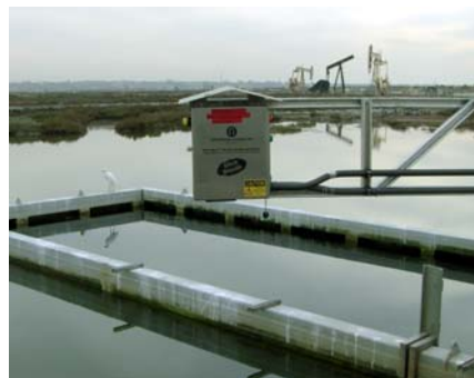
Figures 9, 10 & 11. Remote spill detection system (4-units total) used to automatically control tidal gates and alert personnel to incursion of oil in wetlands/tidelands near production area. Oil producer collaborated with the State of California to safeguard the Bolsa Chica Wetlands, a tidal zone with many valuable indigenous species.
