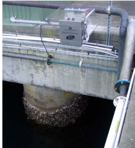
Figure 8. Oil detection sensor on a Navy fuel pier, monitoring for diesel oil on harbor surface in a port setting.
